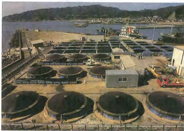
FIG 15 The Hota Fisheries Cooperative, located on the shores of Tokyo Bay near the Tokyo metropolitan area, has built ten circular fish tanks (diameter: 10m) with prefectural grants, and 28 square fish tanks (6m x 6m) strictly with cooperative funding. With these facilities the cooperative cultures 100 tons of bastard halibut annually in addition to culturing or keeping a wide variety of high-priced fishery products such as red sea bream, silver salmon, black sea bream, spiny lobster, sea urchin, abalone, oysters, scallops and top shell, which it then sells to the Tokyo market. Taking advantage of its location just 100km from the enormous metropolitan consumer market, the cooperative seeks to 1) buy young fish from other regions, raise them for about a year and then ship them to market at an appropriate time, and 2) to build up a "Live Fish Center" that keeps live stocks of a variety of high-priced fishery products that can be supplied to the Tokyo market at any time in response to changing market demand.
